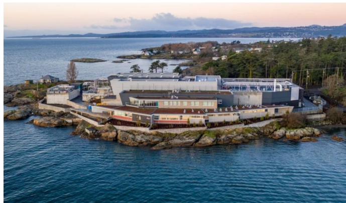
McLoughlin Point Wastewater Treatment Plant Victoria, BC, Canada
